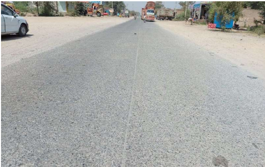
EXISTING ROAD AT KM 44+800 (AFTER LALIAN)
