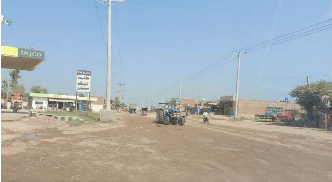
ROAD CONDITION AT KM 7+100
