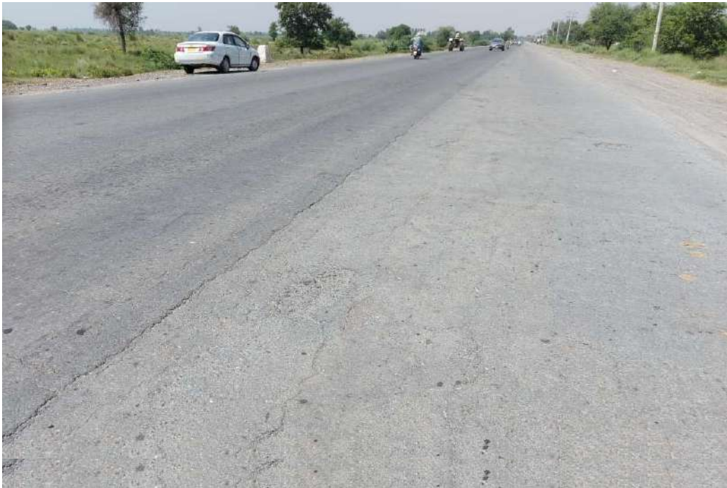
EXISTING ROAD AT KM 38+800
