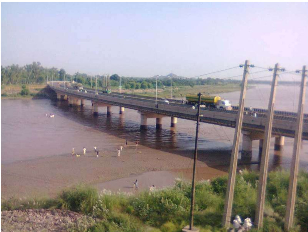
EXISTING DUALIZED BRIDGE ON RIVER CHENAB
