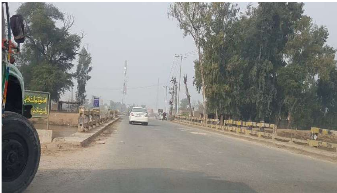
EXISTING 2- LANE CANAL CROSSING BRIDGE (JHANG BRANCH) KM 6+000 (APROX.)
