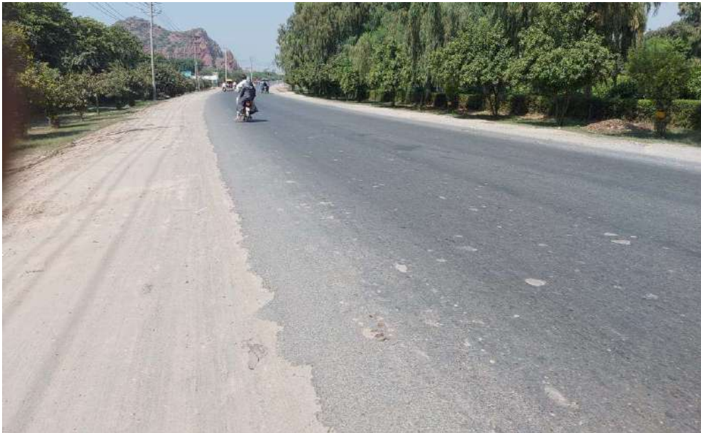
START OF CHENAB NAGAR - SARGODHA SECTION KM 28+300
