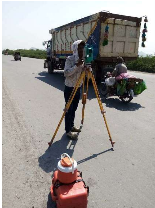
TOPOGRAPHIC SURVEY OF PROJECT AREA WITH TOTAL STATION
